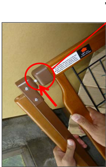
Figure 1. Locking Pin shown above does not lock properly.
